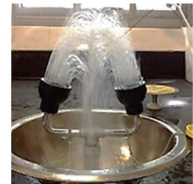
Eyewashes are required for labs operating a BSL-2, though they are often found in BSL-1 labs as well. Eyewashes must be maintained in good working order, activated weekly and tested according to **GS5115: UT Health Science Center Emergency**
