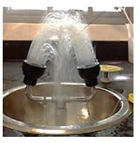
Eyewashes are required for labs operating a BSL-2, though they are often found in BSL-1 labs as well. Eyewashes must be maintained in good working order, activated weekly and tested according to **GS5115**: UT Health Science **Center Emergency**
